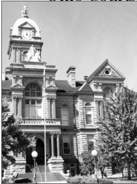
Hancock County Courthouse Findlay
